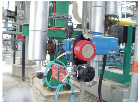
ESD-valve with ValveGuard ensuring customer process safety
