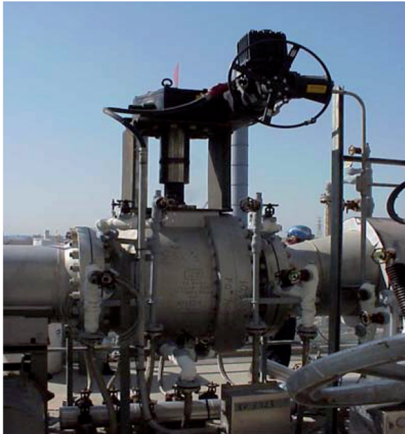
Figure 3. Metso 24" MBV at customer's Coker plant
