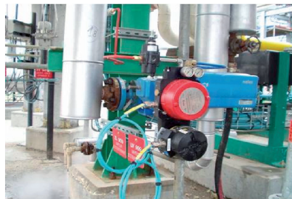
ESD-valve with ValveGuard ensuring customer process safety
