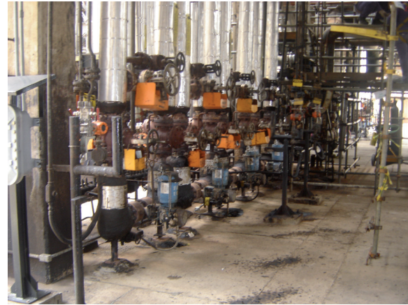
Metso Finetrol valves at customer heater pass flow control
