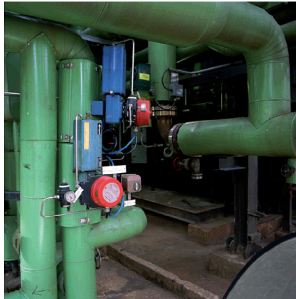
ESD-valve with ValveGuard ensuring customer process safety
