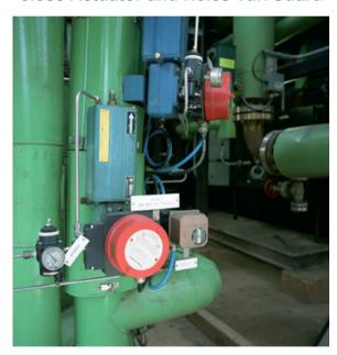
Due to the high oil temperature a smallest leakage may cause a fire. Coke formation takes place in temperatures above 300 °C. This and the corrosiveness of the oil are causing need for more cleaning and maintenance at the pumps and their suction filters than with clean fluids. These operations are to be executed when hot oil under pressure flows in the neighboring piping.
